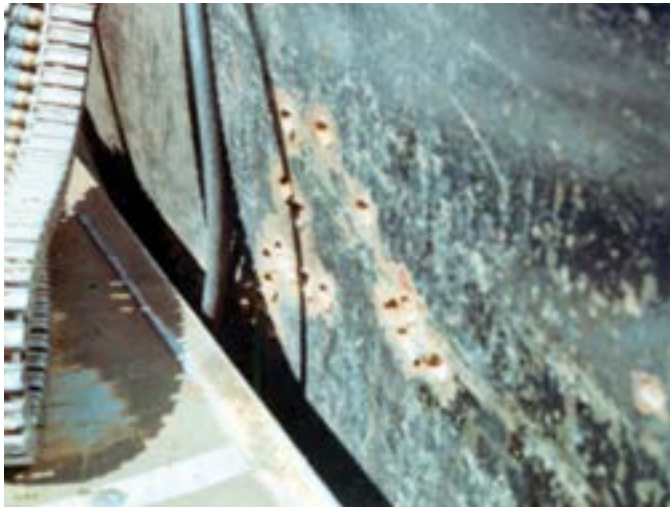
Damage caused by shrapnel bounding off the wall.
